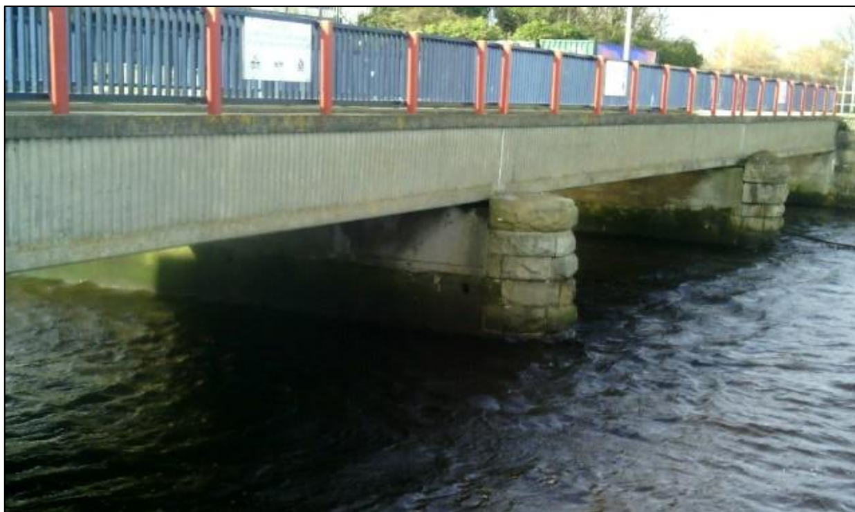
Figure 15 - Road Bridge at Section 16 Looking Upstream
