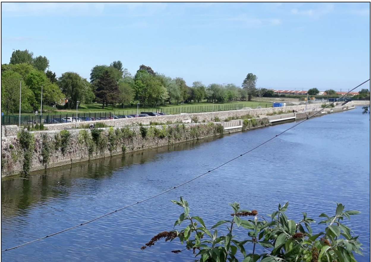
Figure 11 - River Dargle at Cross Section S-6 Looking Downstream
