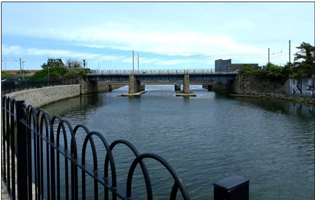
Figure 14 - Railway Bridge at Section 12 Looking Downstream
